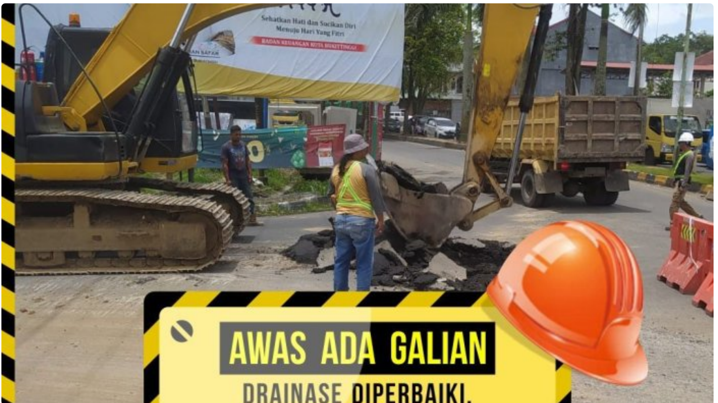
Drainase Diperbaiki, Upaya Pengendalian Banjir By Pass Bukittinggi
